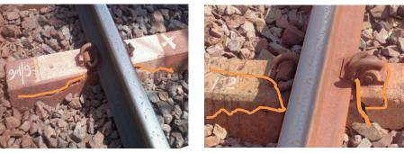
(c) Third Step (Cracks near insert location)
